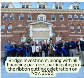
Dezendorf Hall offers 1-bedroom and 3-bedroom affordable apartments within the former college dormitory at Shimer Square in rural Mt. Carroll, IL.
